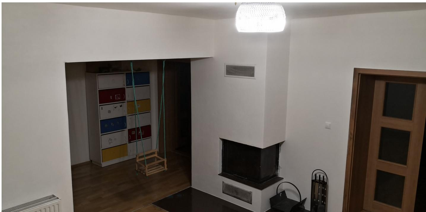
**Led chandelier extinguishing: Model 6** is a simple and cheap room protection system from a height of 2m to 4m! Extinguishing the room has a maximum area of 50 m<sup>2</sup> and a maximum volume of 150 m<sup>3</sup>. Fire extinguishing takes place simultaneously on the area but also the entire volume of the room. It is ideally used for extinguishing spaces with a ceiling height of more than 3,5 m.
