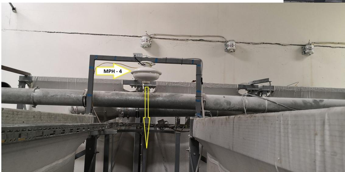
**STOP-FIRE-SAPFIR** autonomous fire extinguishing systems are used for extinguishing all types of electrical equipment. They are designed for extinguishing narrow and long cable ducts, as well as electric transformers and wind power plants up to 40,000 V.
